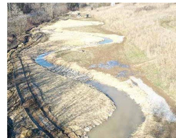
This creek in the Big Bone Watershed is currently being restored. Re-routing a stream to a more natural state can improve water quality and wildlife habitat.
