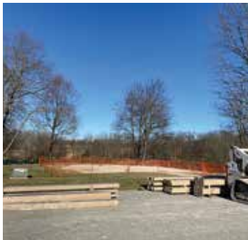
New shelter under construction at England-Idlewild Park
